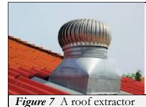
Figure 7 A roof extractor
