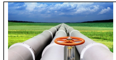
Figure 24 Over-ground petroleum pipes laid over terrain prone to freezing in winter
