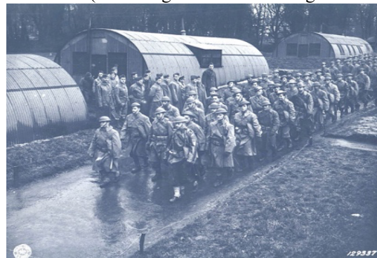
Figure 35 Vintage picture of a Quonset hut 35 from the second World War. Note the self-supporting roof and door at the gable end. These huts were not designed for industry and afford very little ventilation possibility.
