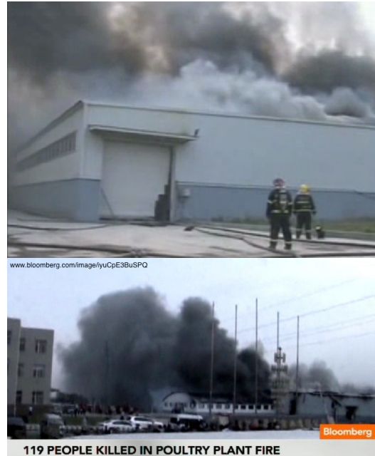
119 PEOPLE KILLED IN POULTRY PLANT FIRE Figures 3, 4 The upper picture shows a probable packing material receipt gate (D1 of figures 7, 10). The brick wall in figure 14 is apparently behind the sheet steel-dado wall seen here. The bottom picture, taken from across the highway near the main gate area, shows the admin building on the left.
