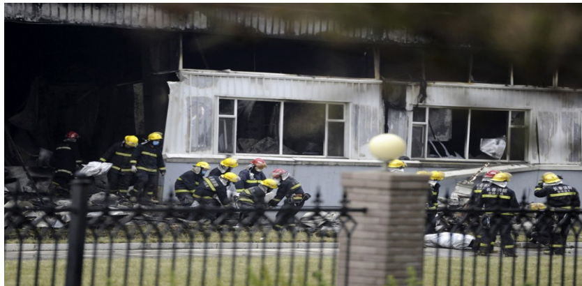
Figure 26. This picture gives a good idea of the roof height at the eaves on the south end – some 7-8 metres. It also gives a good view of the prefab construction with fixed windows. Notice the vertical smear line left by escaping smoke. This line marks the joint between two adjacent prefab panels. The north wall comprises prefab panels alternating with sandwich panels, but the south end has only prefab sections.
