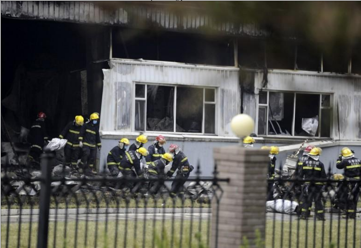
Figure 13. This picture gives a good idea of the roof height at the South end –some 6-7 metres. It also gives a good view of the prefab construction with fixed windows.
