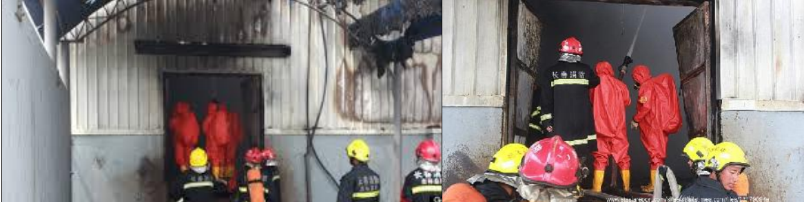
Figure 11, 12. The East side of the building (the rear in Figure 5), serves for arrival of live birds. In the above pictures you can see rescue attempts being made from one such bays after the firemen have knocked open the door from outside. The roof of the bay shelter (Figure 11) is gone, probably blown off and the heat signature on the sheet metal wall of Figure 12 shows that the insulation was on fire from within. Notice that this bay has a big plinth.
