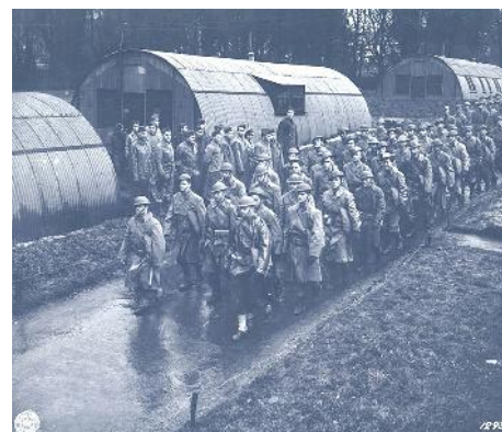
Figure 16: A Quonset hut from the Second World War. Note the self supporting roof and door at the gable end
