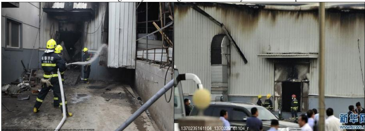
Figures 18, 19 The first picture shows firefighters located in one of the bays formed by the several abutting sheds and structures to the East end of the main process area. The other picture, taken at the West end, before the entire wall was torn down as part of rescue efforts (Figure 5) shows some signs of fire and - a collapsed roof-gutter. This forms two possible emergency exits, one of them added as an afterthought – the height, shape and absence of protection against rain at this doorway suggesting that it opens not into the process area, but into an internally located utility area..
